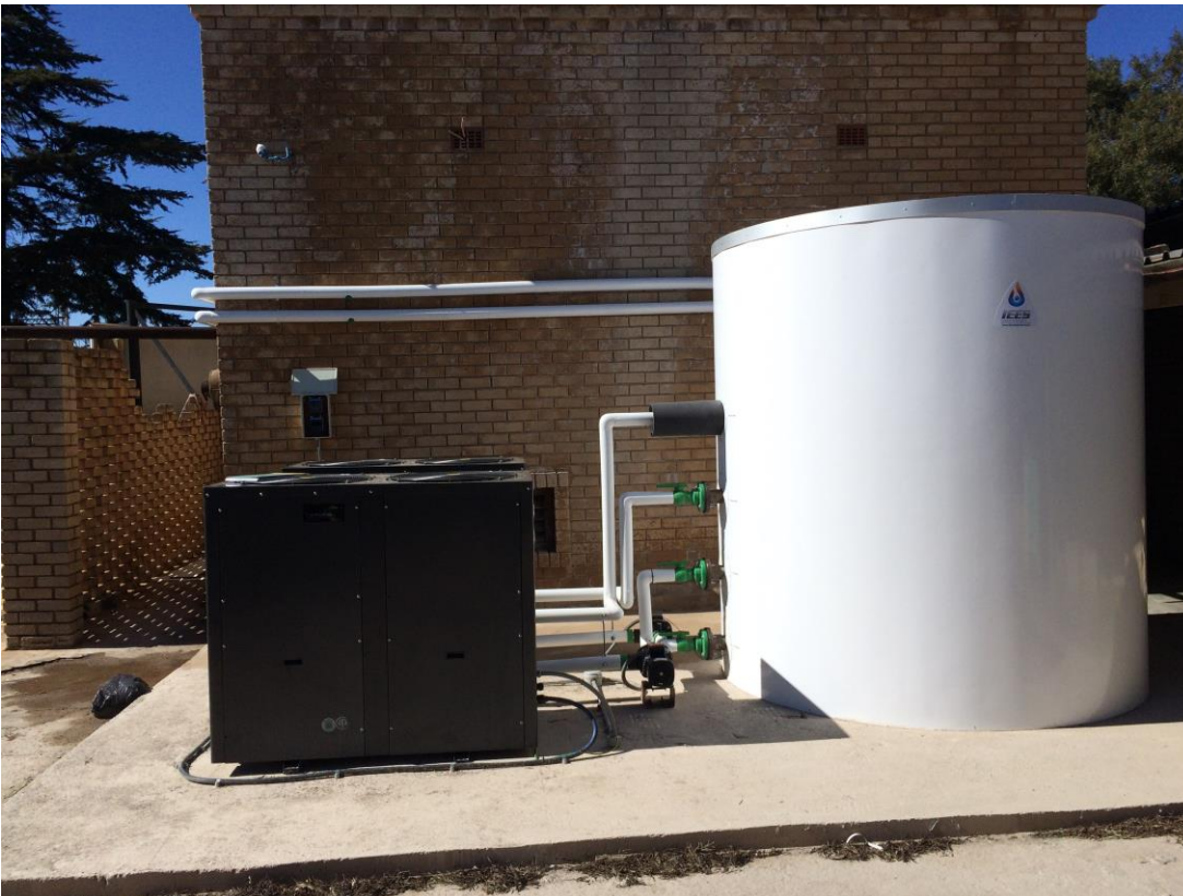
Complete installation with well insulated ring main resulting in a 63.04% saving on electricity.
