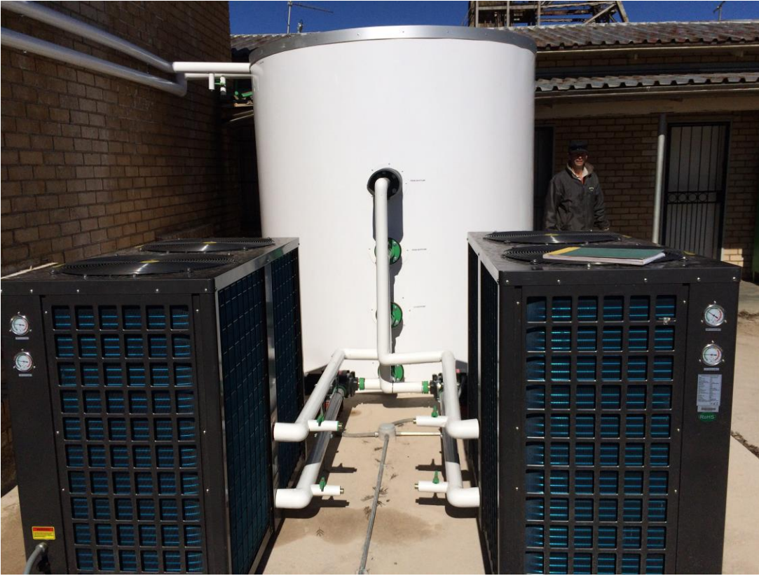
New 8000L fiber glass heat exchange boiler fitted to 2 x 45 kWatt heat pumps
